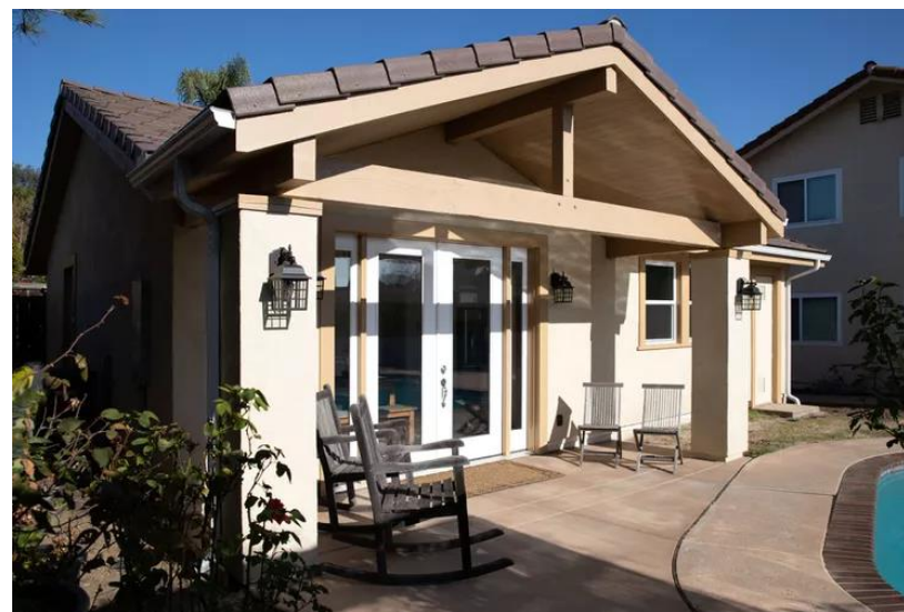
Monterey Bay, California ADU. Source: County of Santa Cruz My House My Home Program .
