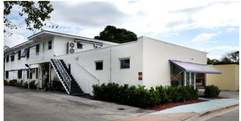
Proposed multi-tenant housing project in Delray Beach. Photo courtesy of the Sun Sentinel.
