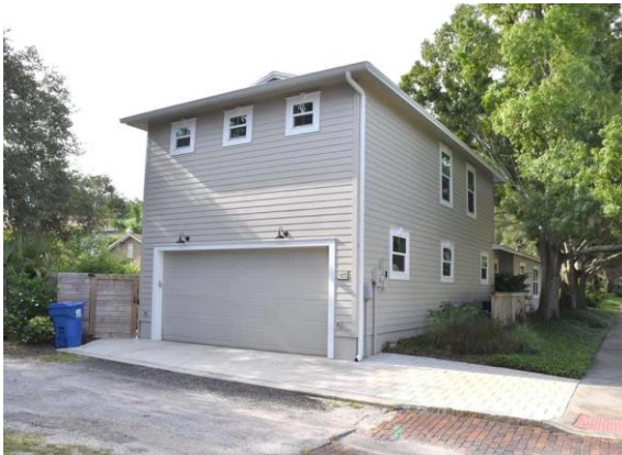
Above-garage accessory dwelling unit in St. Petersburg, FL. Source: Sun Bay Builders.
