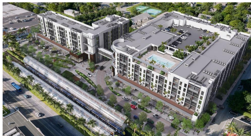
The Horizon of Oakland Park final rendering of TOD mixed-use project. Rendering courtesy of City of Oakland Park.
