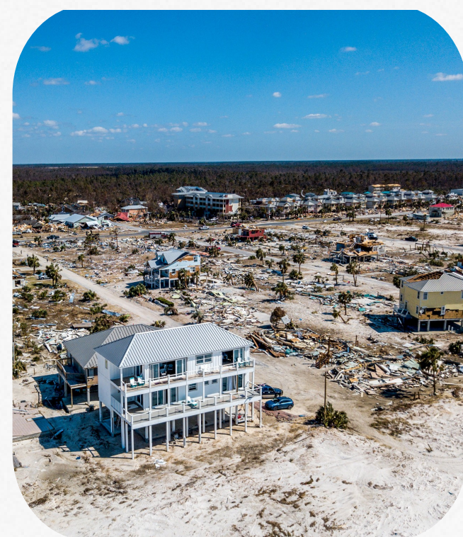
Mexico City, Florida after Hurricane Michael
